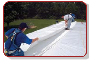
Prefabricated Roofing System
